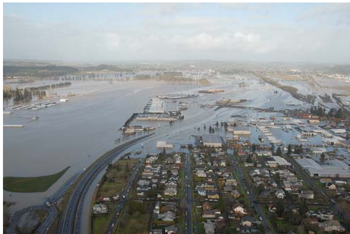
An aerial photo showing the flood waters over I-5 in Chehalis on December 4, 2007. Source: WSDOT
